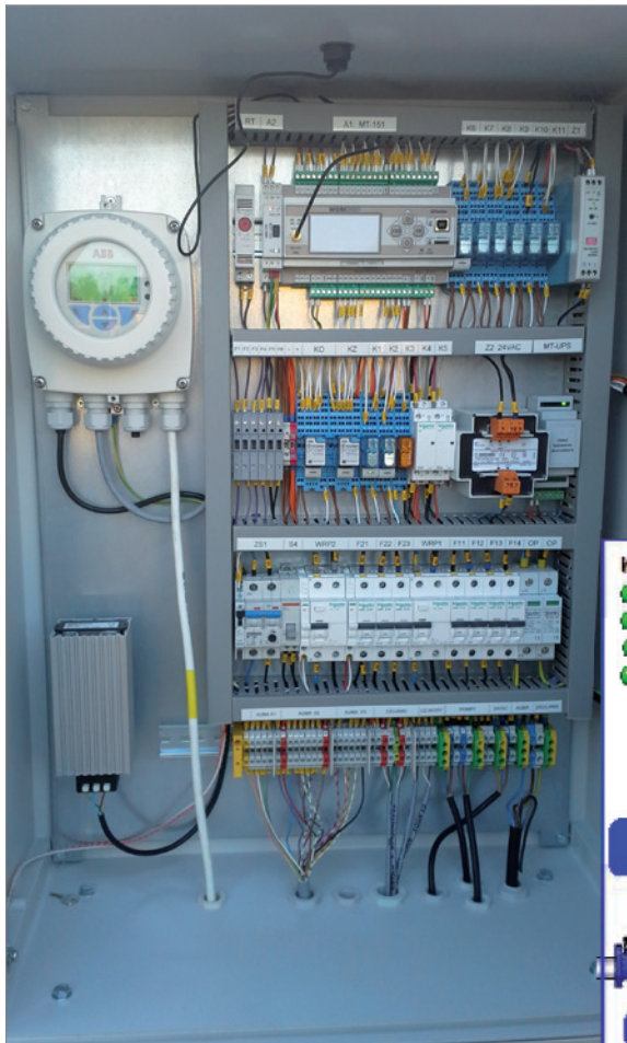
MT-151 HMI module controlling dampers in measuring chambers of clean water pipes
