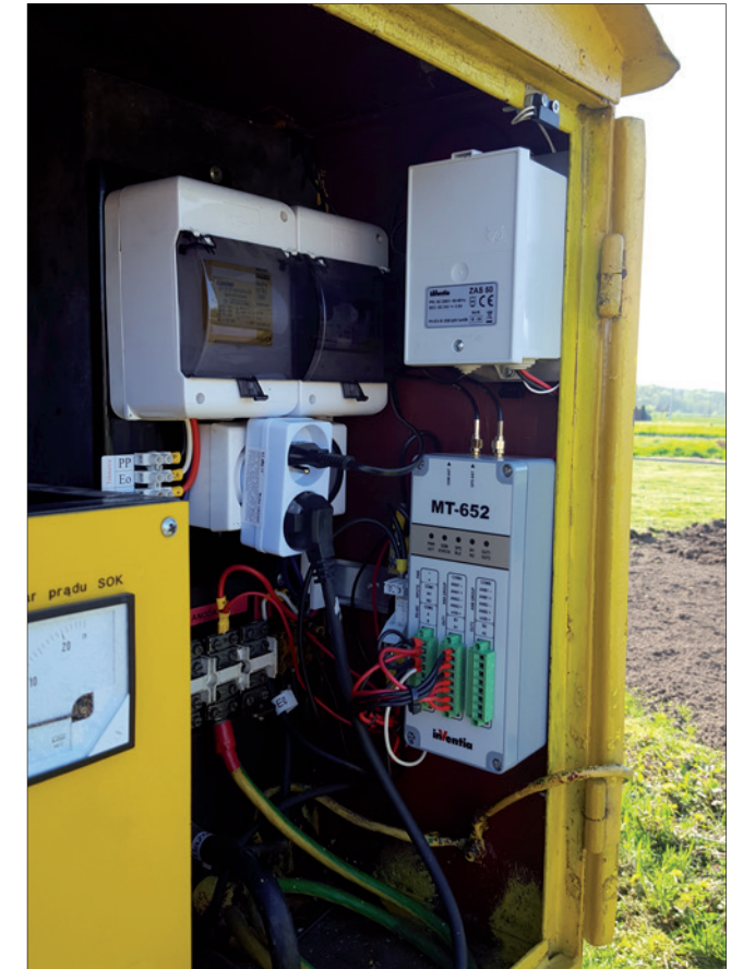
View of the MT-652 module installed in a transformer-rectifier cabinet
